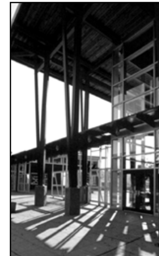
Redmond High School Photovoltaics, Lake Washington School District
