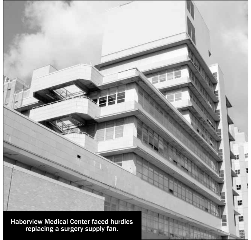
Use the strictest clean-site precautions in critical areas such as surgery rooms.
