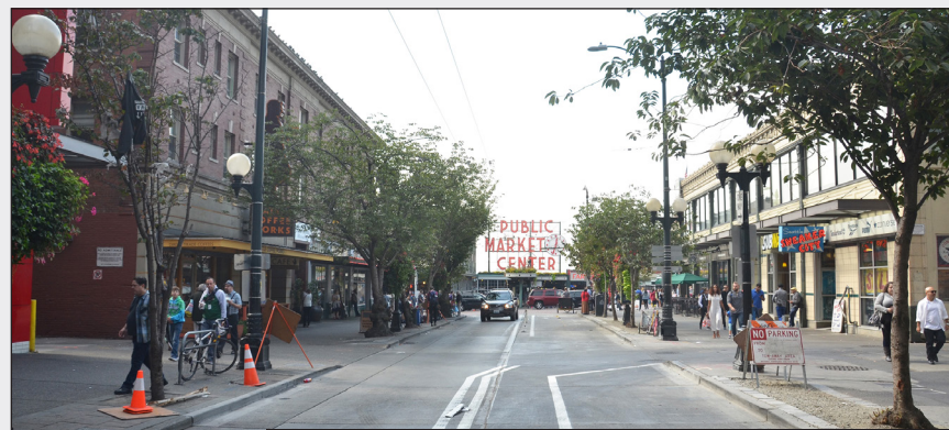
Pike Street would be reconfigured as a shared street between Pike Place Market and Second Avenue.
