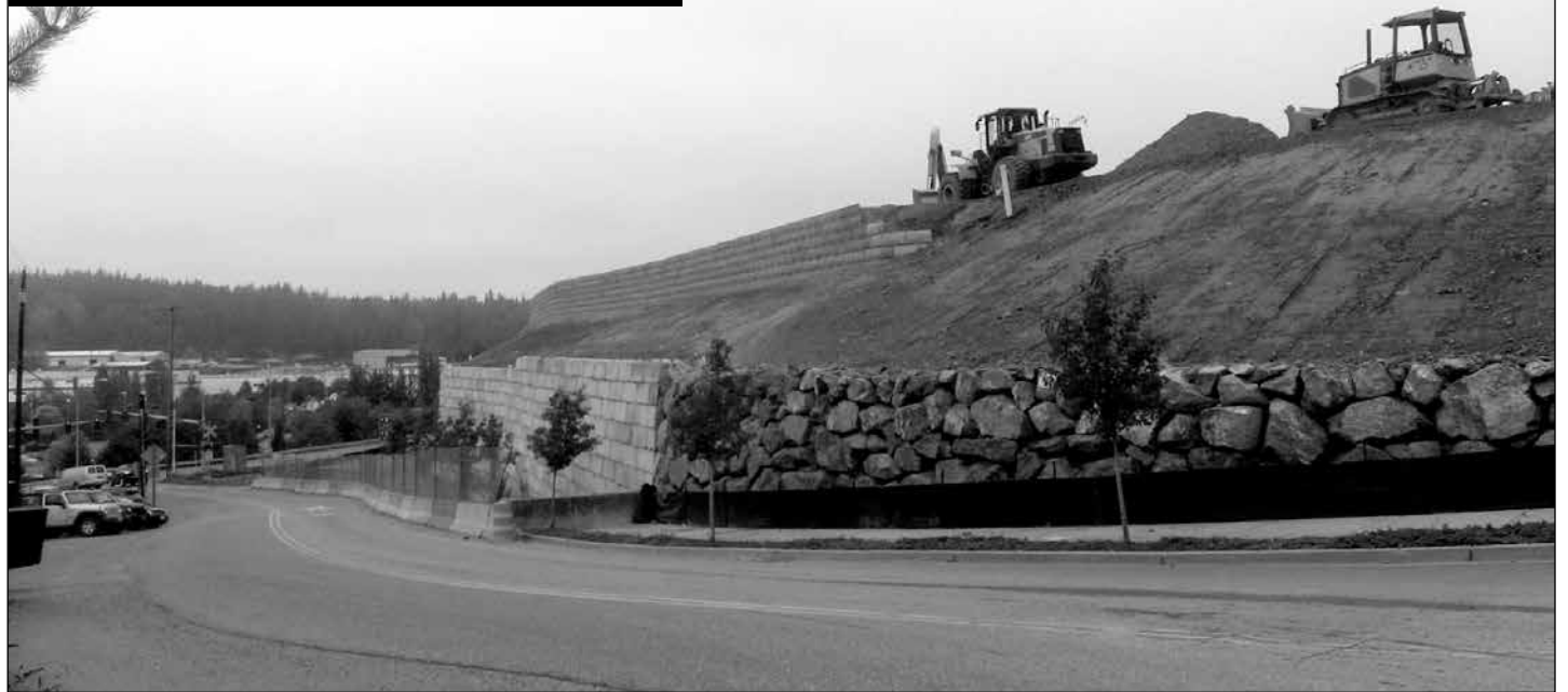
PHOTO FROM DONOVAN BROTHERS CONSTRUCTION
