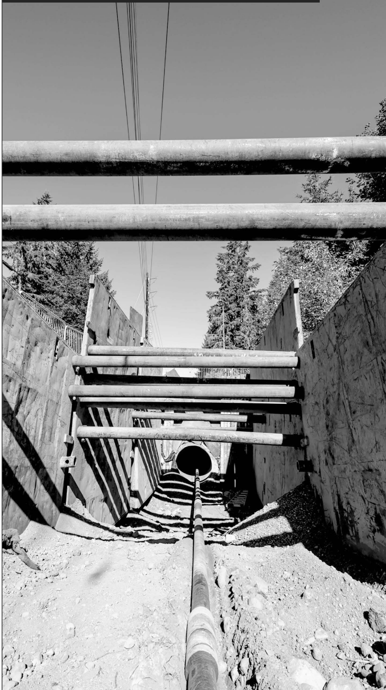
PHOTO COURTESY OF IMCO GENERAL CONSTRUCTION
