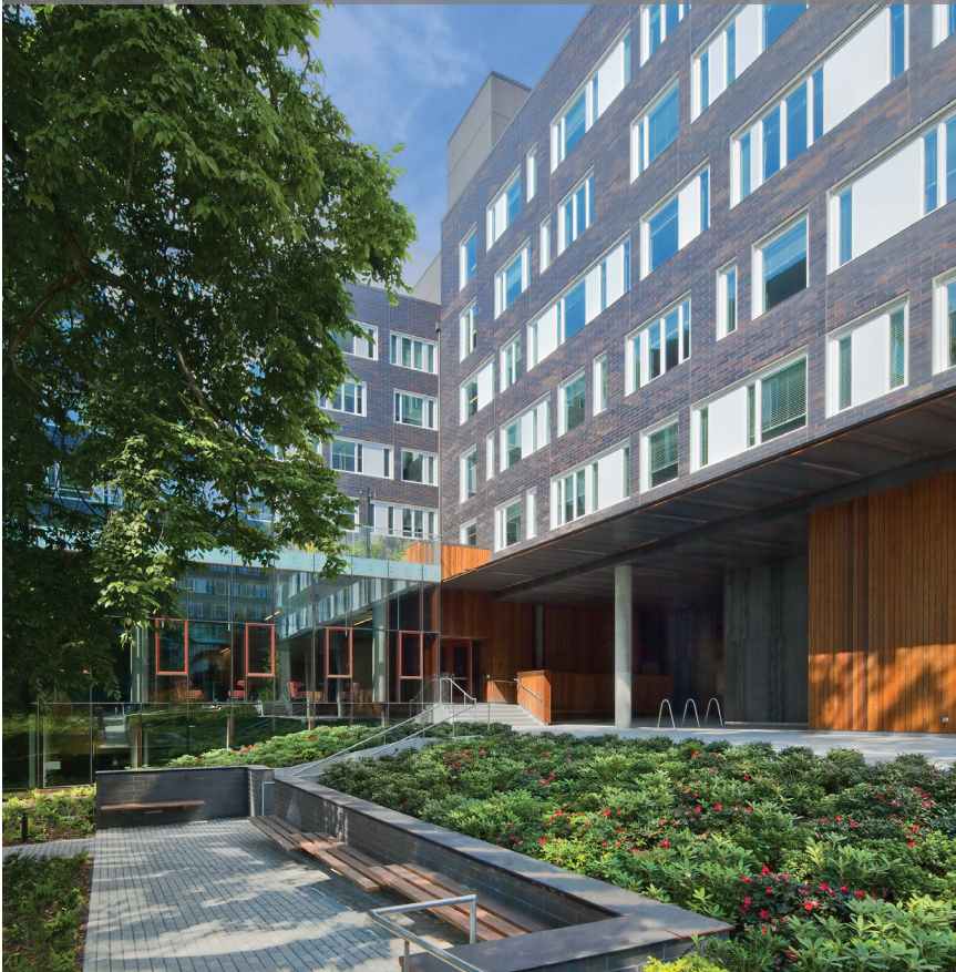
UW Elm Hall LEED Gold
