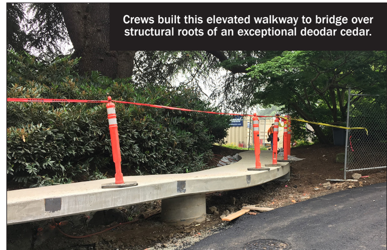
The finished walkway caused minimal damage to structural tree roots.
