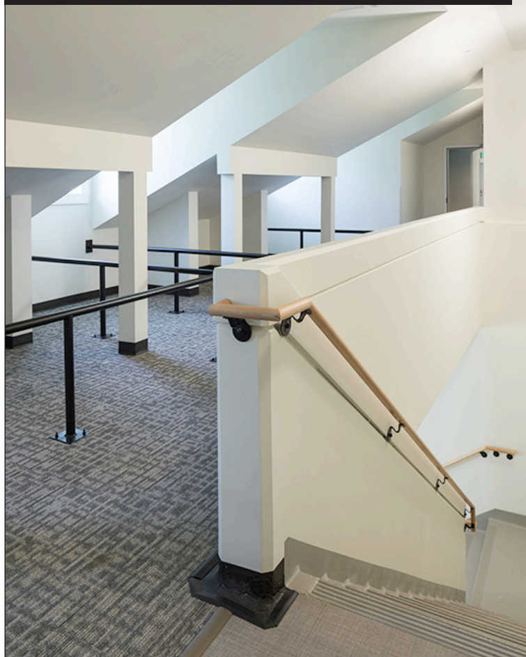
The nearly 100-year-old Sand Point Building 9 presented a multitude of obstacles when turning it into 148 affordable housing units, community services, and commercial tenant spaces.
