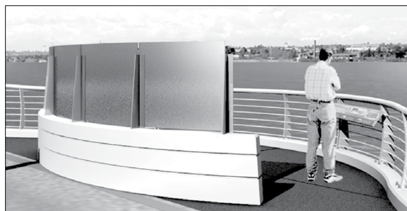
Belvederes offer cyclists and pedestrians places to stop and admire the views. Windscreens shield visitors from highway noise and wind.
