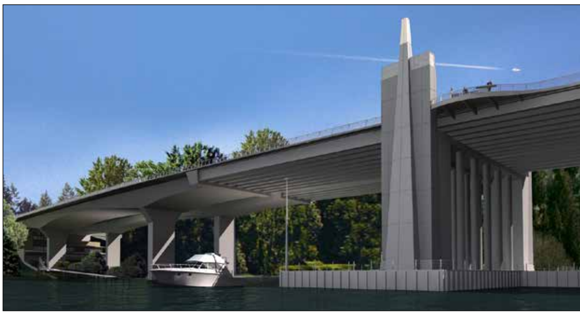
Sentinels as tall as 115 feet serve as a gateway to the floating bridge.
