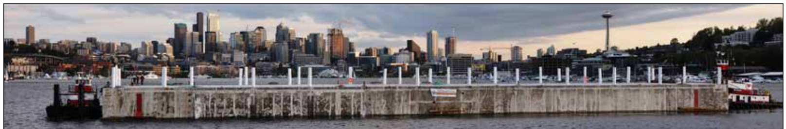
Contractors built all the bridge's jumbo pontoons in Aberdeen, then hauled them to Lake Washington.
