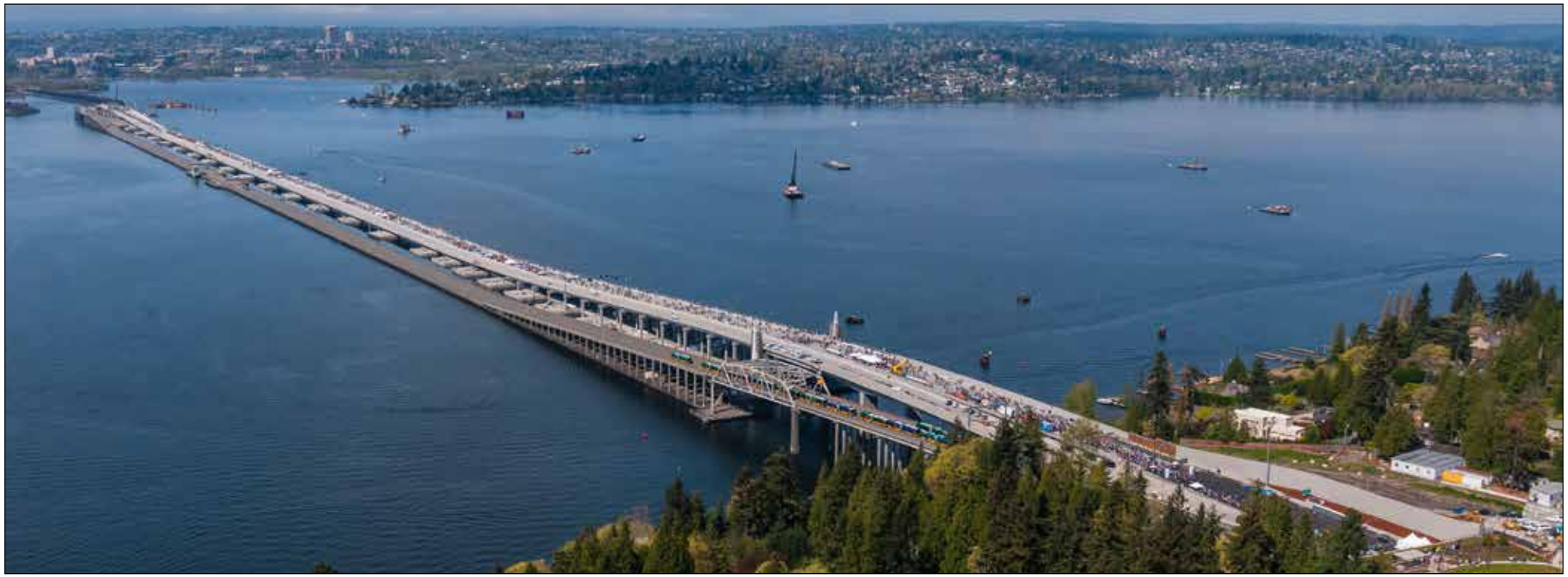
The new floating bridge rests atop 77 concrete pontoons, the largest of which weigh 22 million pounds.
